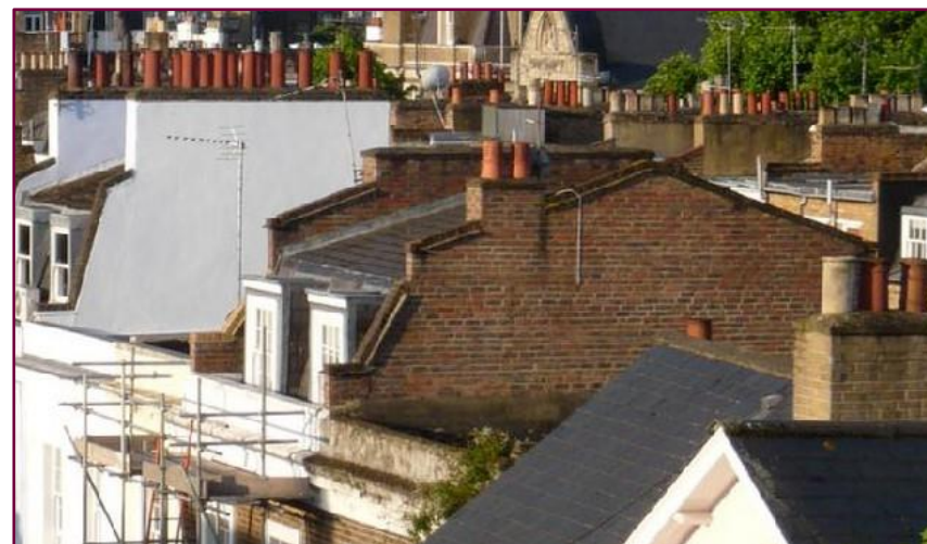
Double pitched mansard roof extension in our area.
