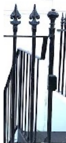
Talbot Road North railings
