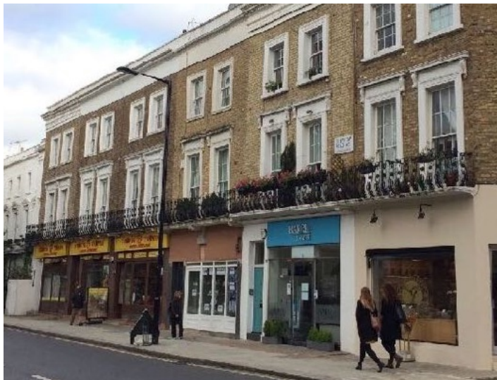
Shops on Chepstow Road
