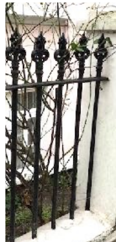
Talbot Road South railings
