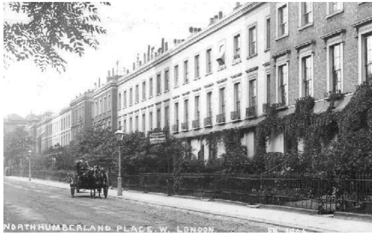
The original Northumberland Place railings had spear or fleur-de-lys shaped heads, and a secondary rail and dog bars at the base.
