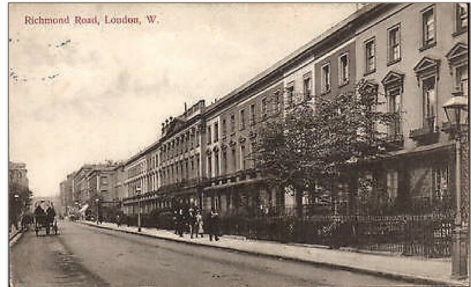
East side of Chepstow Rd. (formerly Richmond Rd.) at end of 19th c. showing central pavilion with pediment and flanking balustrades. These would have been stone coloured render.
