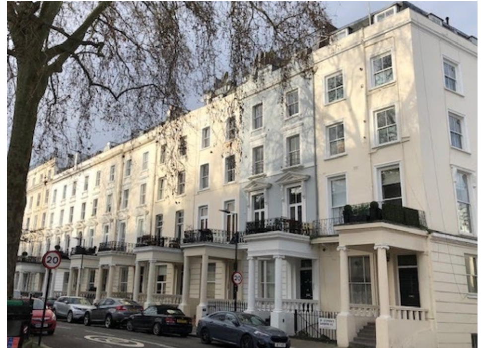
Shown above, eight houses on the north side of St. Stephen's Square with mansard roof extensions are out of step with those to the left.
