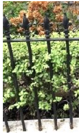
Modern Northumberland Place railings
