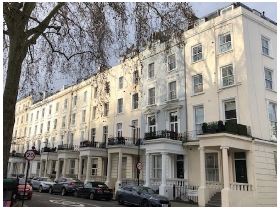
Shown above, eight houses on the north side of St. Stephen's Square with mansard roof extensions. On the left, the top storey has been created by extending the principal elevation upwards.
