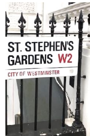
St. Stephen's Gardens South railings
