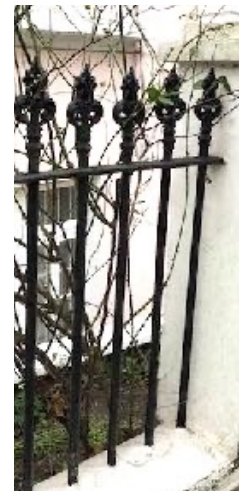
Talbot Road South railings
