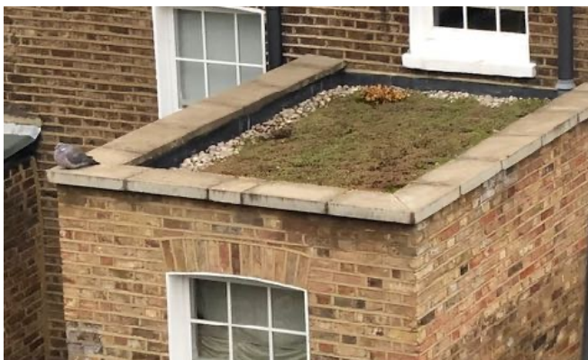
Sedum roof on a rear extension in our area helping to address climate change.
