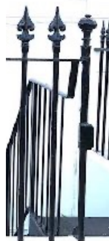
Talbot Road North railings
