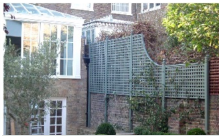
Trellis for privacy - above 2 m high requires planning permission.
