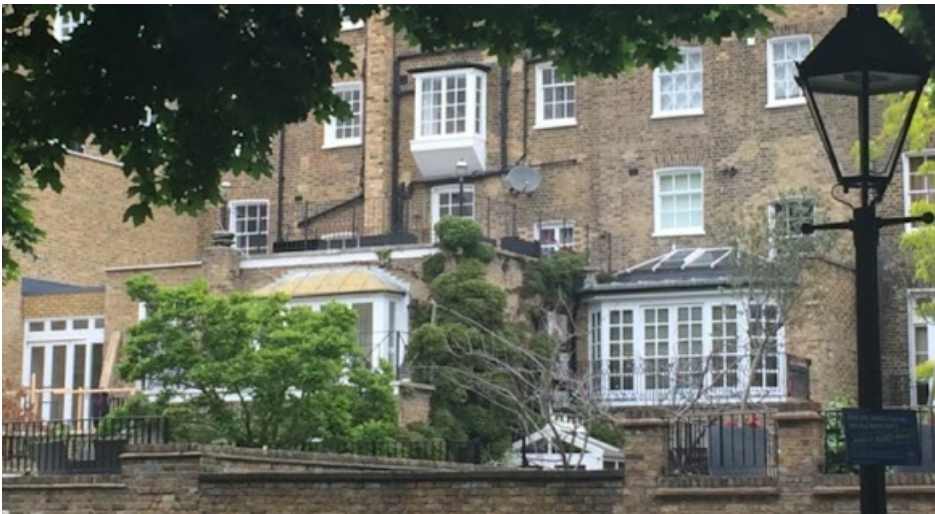
Above, backs of houses in another Westminster neighbourhood with a variety of conservatories, roof terraces, oriel windows and infill extensions.
