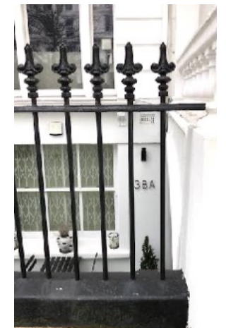
St. Stephen's Gardens North railings
