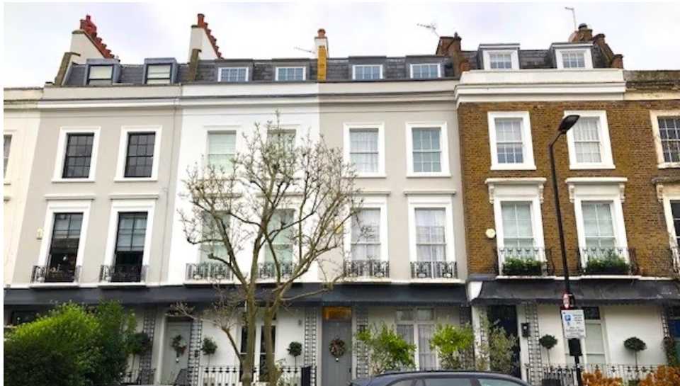
Photo at left from Northumberland Place shows earlier double pitched mansards on each end with two later flat topped mansards in the centre and gaps to the left where mansards have been refused - a consequence of inconsistent planning policy implementation over time. Darker paint finishes on the mansard windows at far left help them to read as part of the roof structure.
