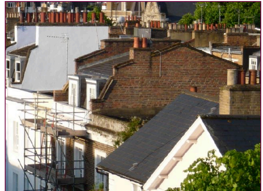
Double pitched mansard roof extension in our area.
