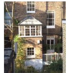
At right, extension with lightweight 3-sided lantern on top storey.
