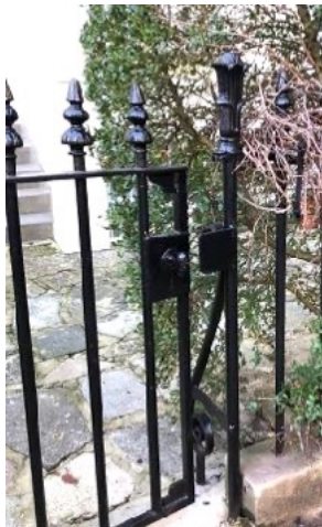
Artesian and Chepstow Road railings
